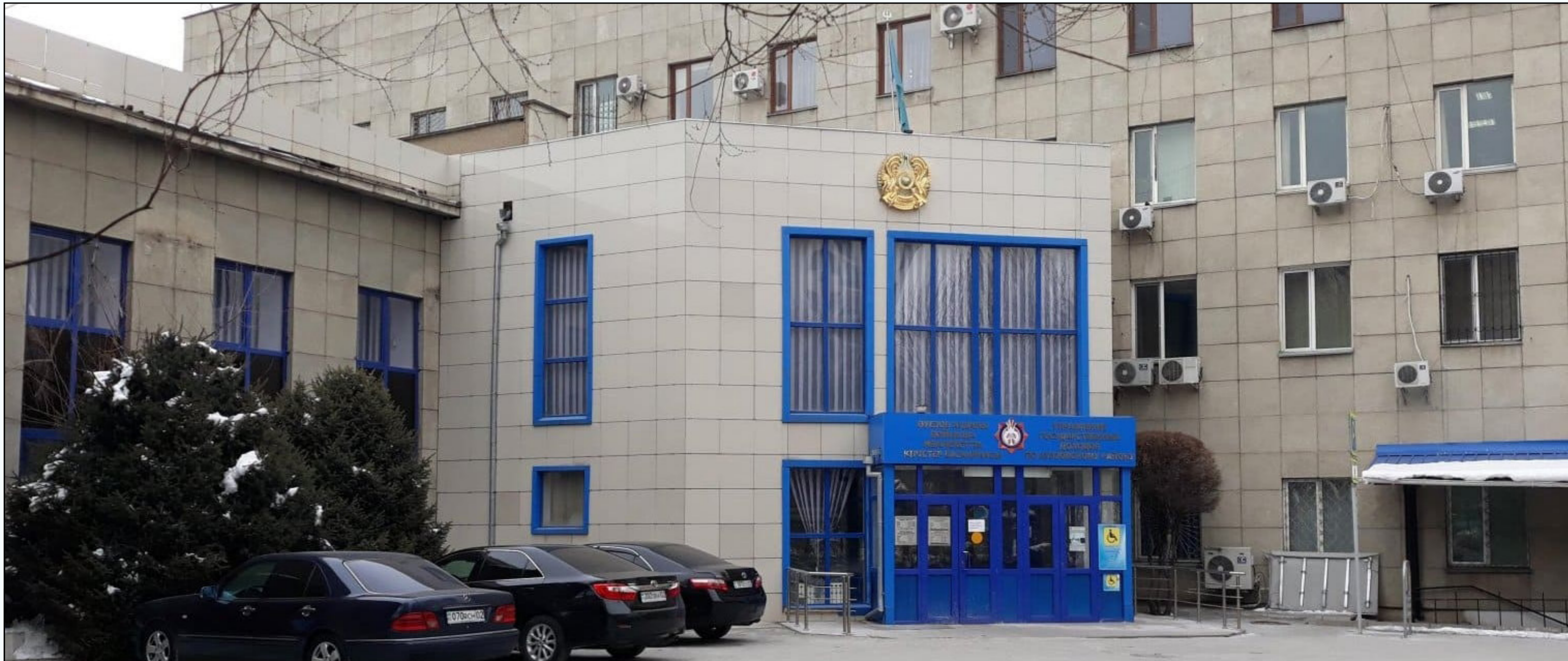
A tax inspectorate office in Almaty.
